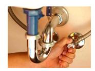
For drain leaks, you can save us a trip by attempting to tighten the connections for the trap under the sink.
