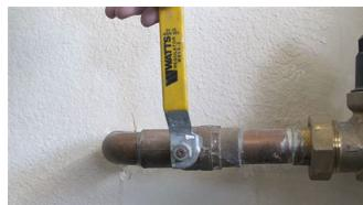
Should you find a leak, turn off water at the furthest point along the line to isolate it. Work your way back to the main valve until it stops. **IF WATER IS GUSHING INTO YOUR HOME - TURN OFF THE MAIN VALVE IN THE HOUSE THEN THE SHUTOFF AT THE STREET IF POSSIBLE AND NOTIFY US IMMEDIATELY.**
