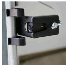
A broom, trash can or even dirt on the lens will cause this condition. It is also not uncommon for one of the beam transmitter/ receivers to be kicked or knocked out of alignment. Just a push to adjust its position or angle is enough to fix the problem. The light will usually be on when it senses a clear beam and off when it's blocked. Some have a yellow and green scheme.
